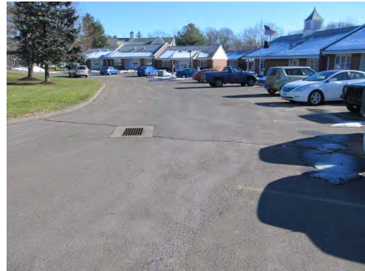
Asphalt paving in parking area in generally good condition – Crackfilling / sealcoating / striping needed in near-term
