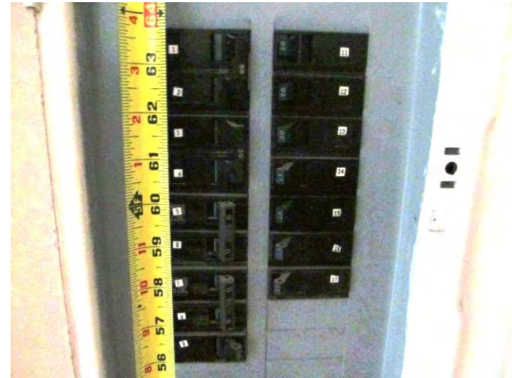
Some circuit breakers in panels at handicap accessible units exceed reach range limits
