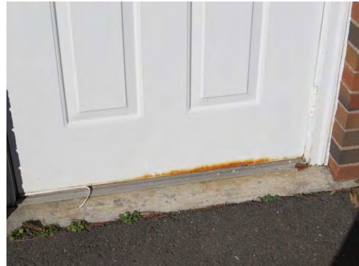
Minor surface rust at bottom edge of service door
