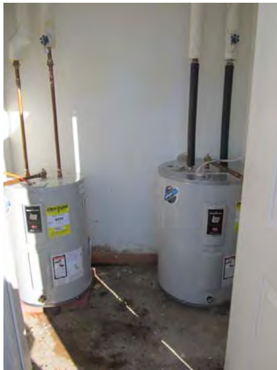
Typical, individual, electric-type domestic hot water tanks that serve each unit
