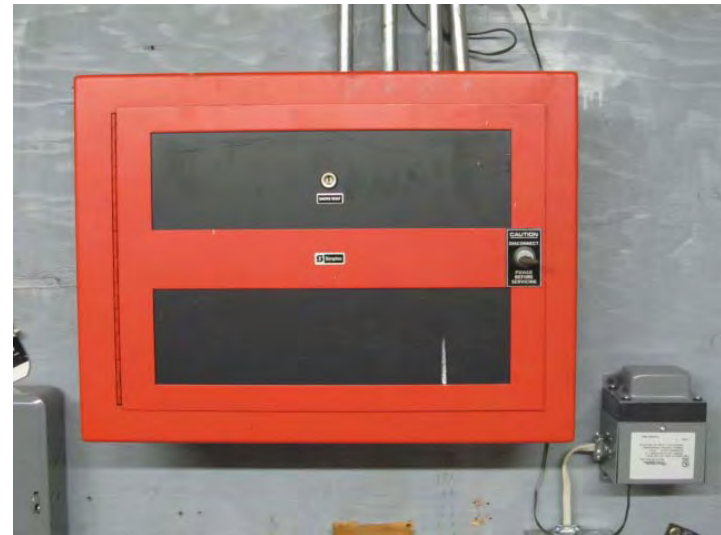
Original fire alarm control panel has surpassed its expected useful service life
