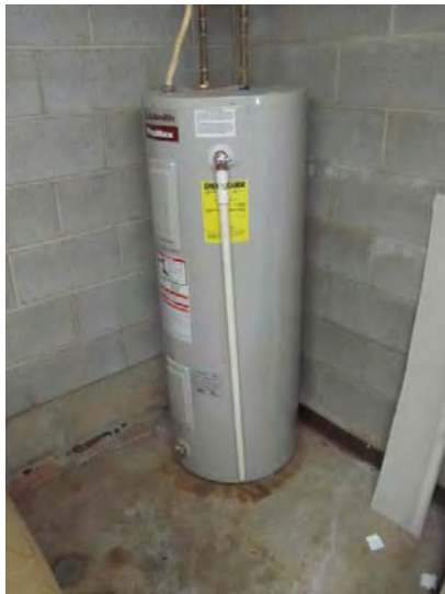
Newer electric-type tank that serves domestic hot water needs at community spaces
