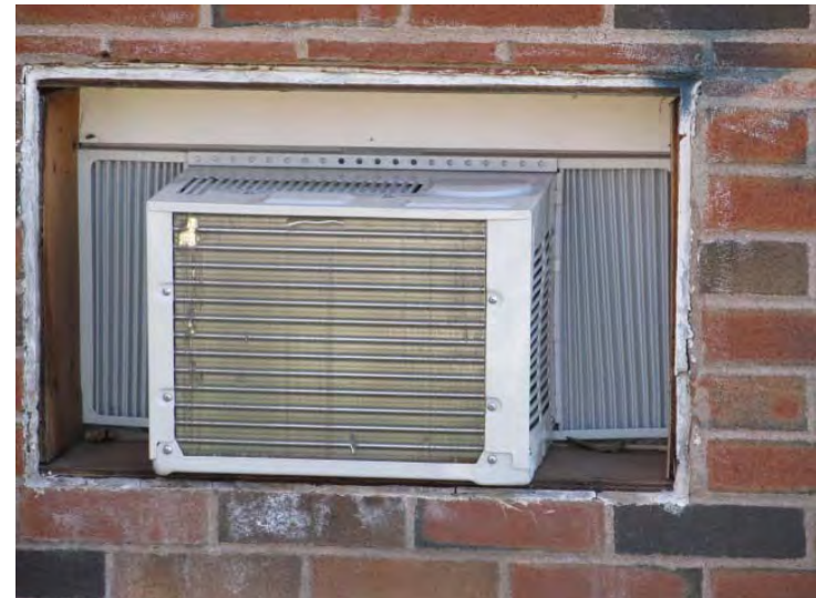
Each unit has a sleeve to accommodate a resident-supplied air conditioner – Note sleeve size compared to air conditioner size
