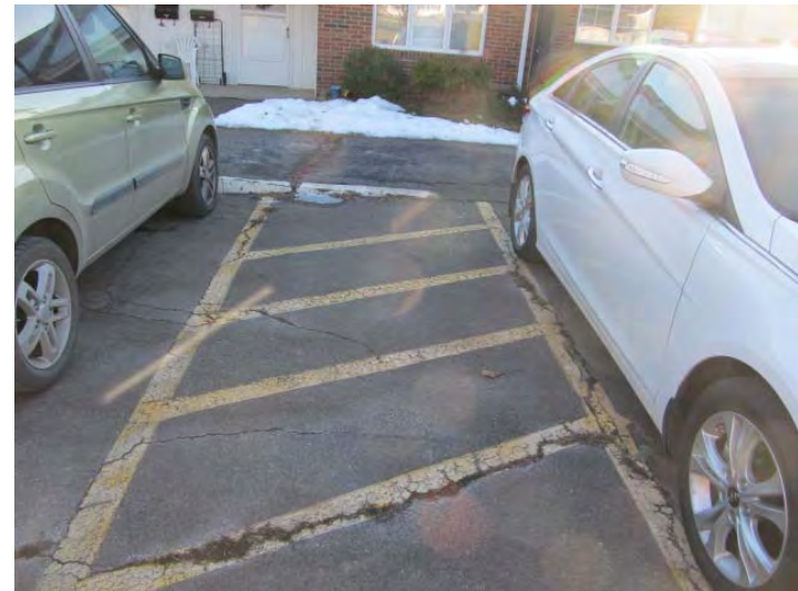
Curb ramp near Units 25 and 26 lacks necessary flared sides for handicap accessibility compliance
