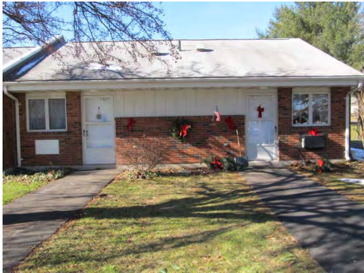
Unit entry and storm doors in good condition at the present time – Original windows are approaching the end of their expected useful service lives
