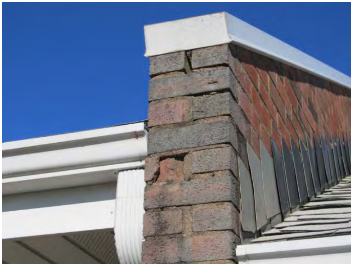
Brick veneer between building segments exhibits areas of cracks, mortar loss, and shaling/spalling
