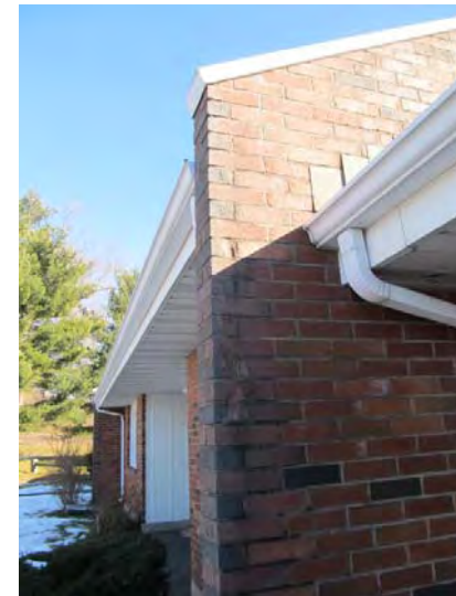
Side view of brick veneer on wall between building segments with worn brick and mortar evident
