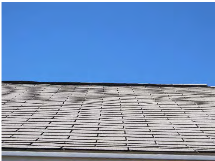
Typical roof surface with three-tab shingles – Some age-related wear beginning to show
